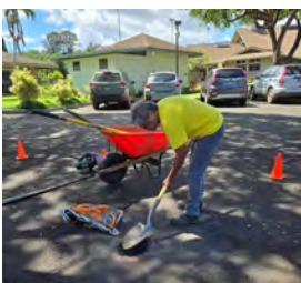
Project 3: repair the parking lot pavement
